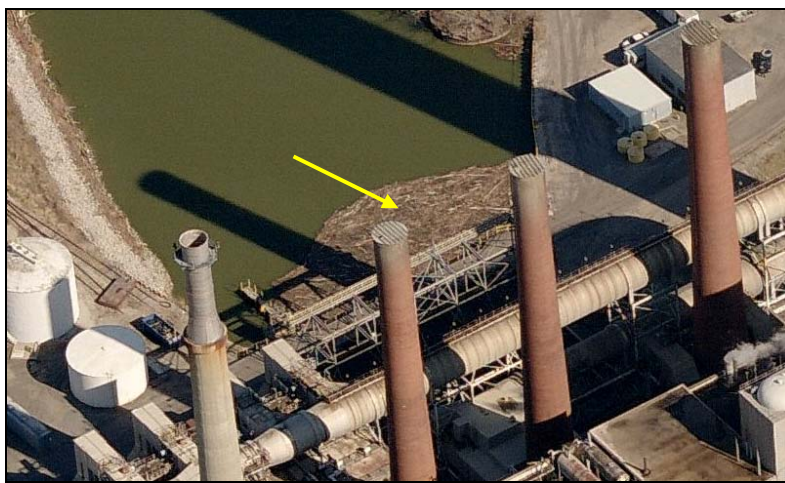
Figure 6. Buildup of Large Debris at CWIS
