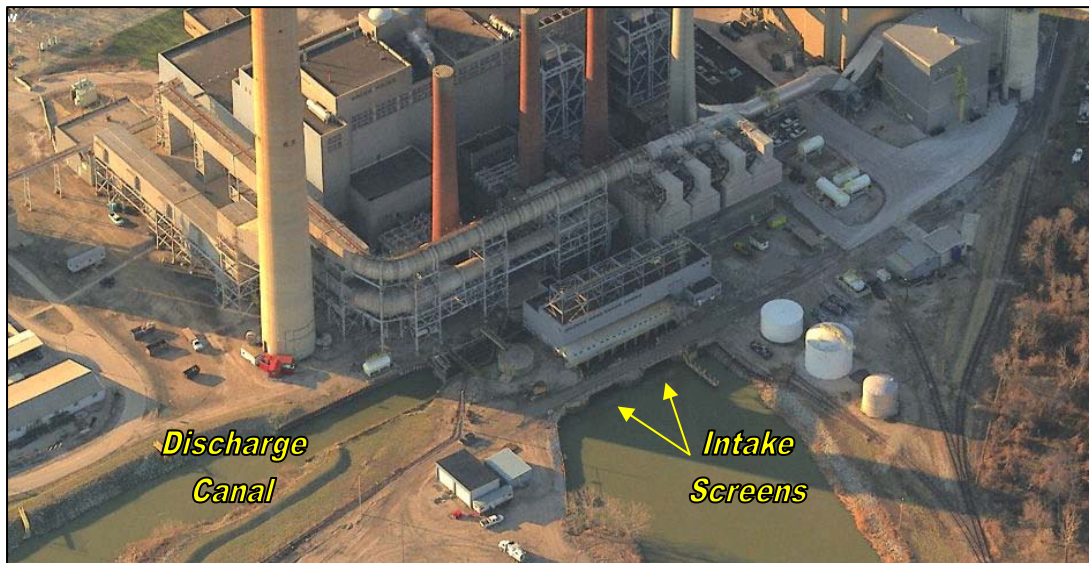
Figure 3. Intake and Discharge Locations
