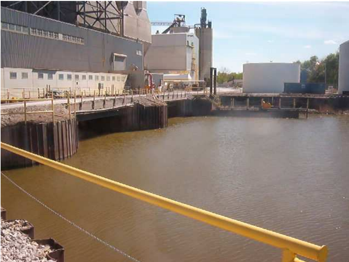
Figure 1.2 Intake at the Bay Shore Power Plant
