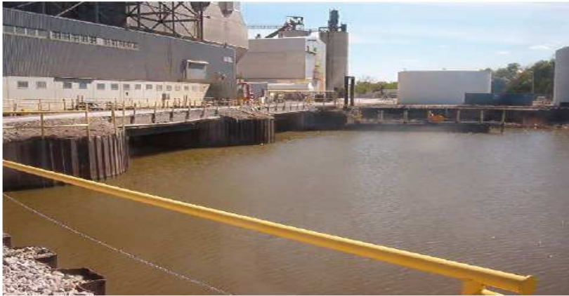
Figure 2. Intake at the Bay Shore Power Plant
